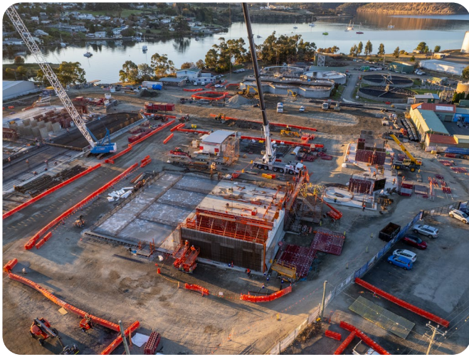
Selfs Point major concrete structures
