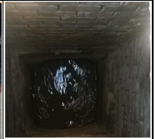
TOPSIDE VIEW OF MANHOLE
