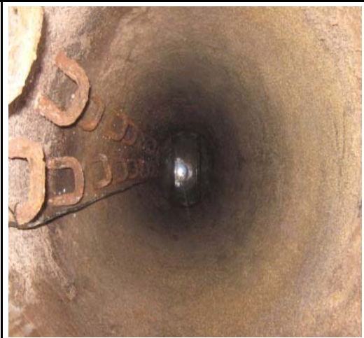
TOPSIDE VIEW OF MANHOLE
