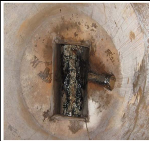
TOPSIDE VIEW OF MANHOLE
