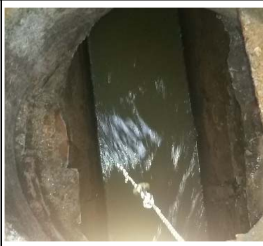
TOPSIDE VIEW OF MANHOLE
