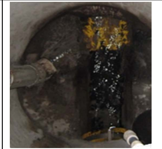
TOPSIDE VIEW OF MANHOLE
