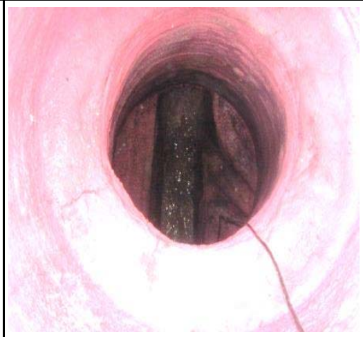
TOPSIDE VIEW OF MANHOLE
