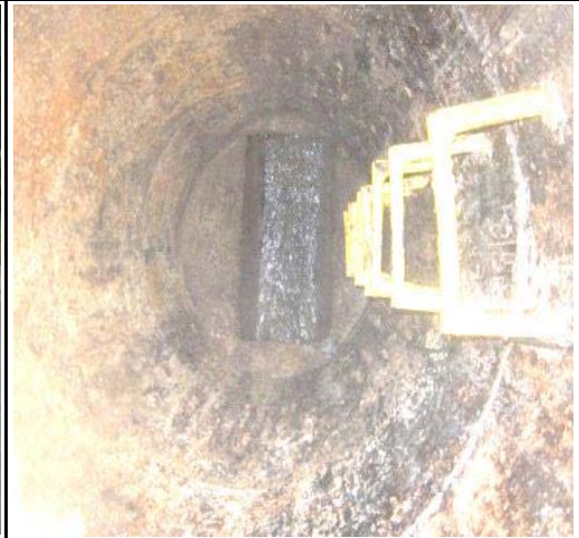
TOPSIDE VIEW OF MANHOLE
