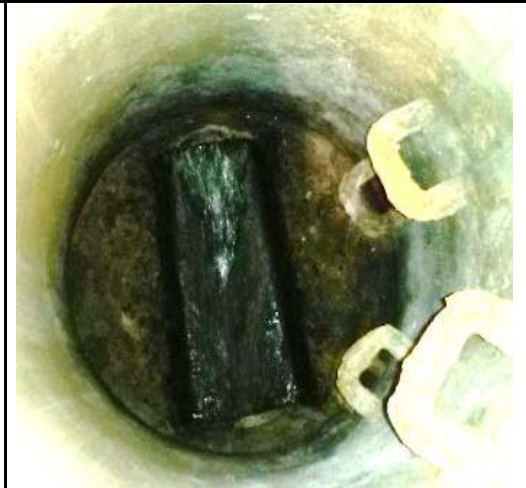
TOPSIDE VIEW OF MANHOLE
