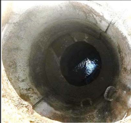
TOPSIDE VIEW OF MANHOLE
