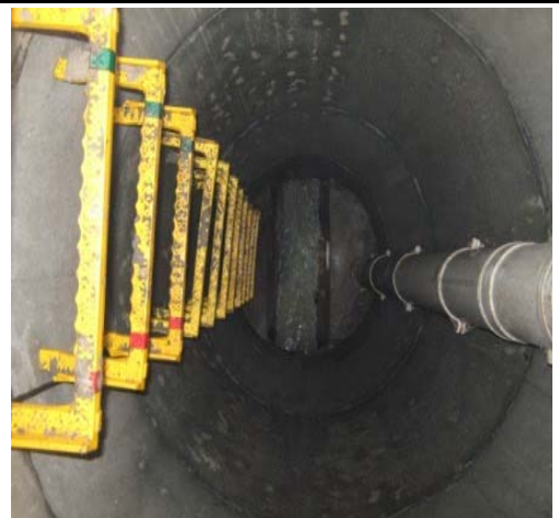
TOPSIDE VIEW OF MANHOLE
