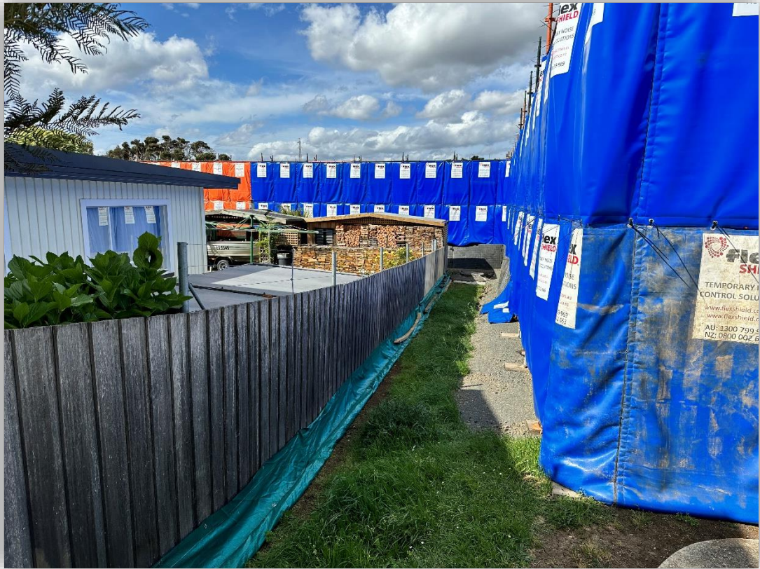
Figure A-3: Photograph of a temporary noise barrier system (taken by Tarkarri Engineering).
