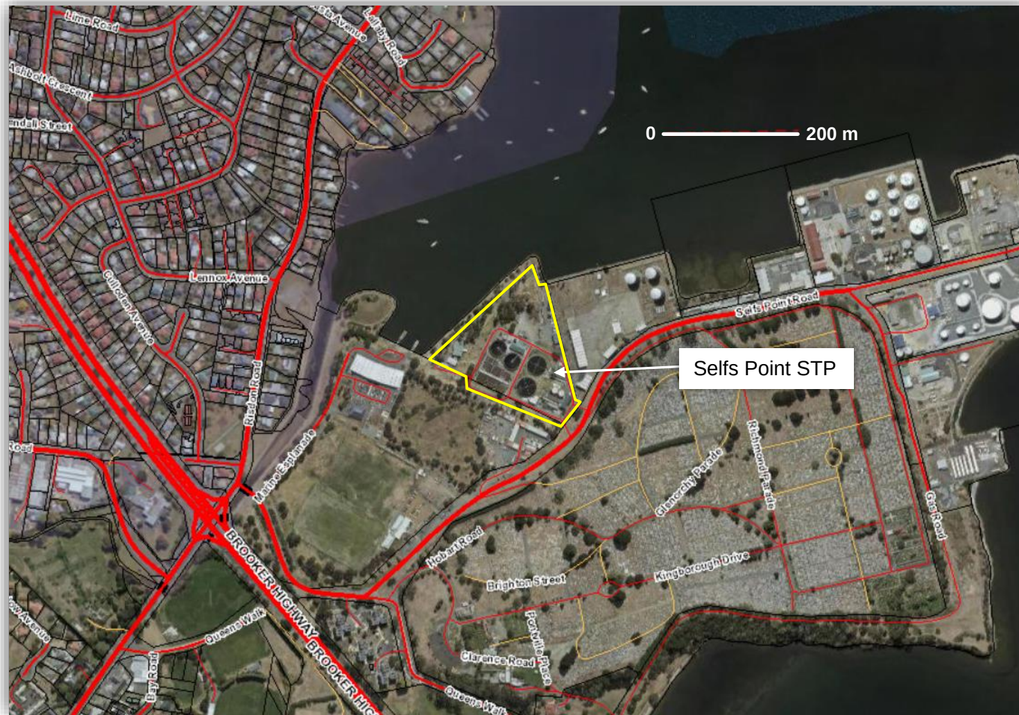
Figure 2-1: Aerial view of existing Selfs Point STP and surrounds.
