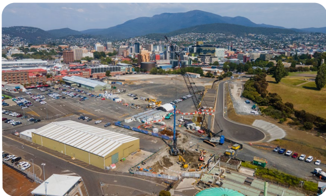
Macquarie Point construction site
