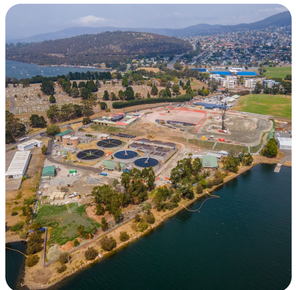
Construction of the new Selfs Point Sewage Treatment Plant
