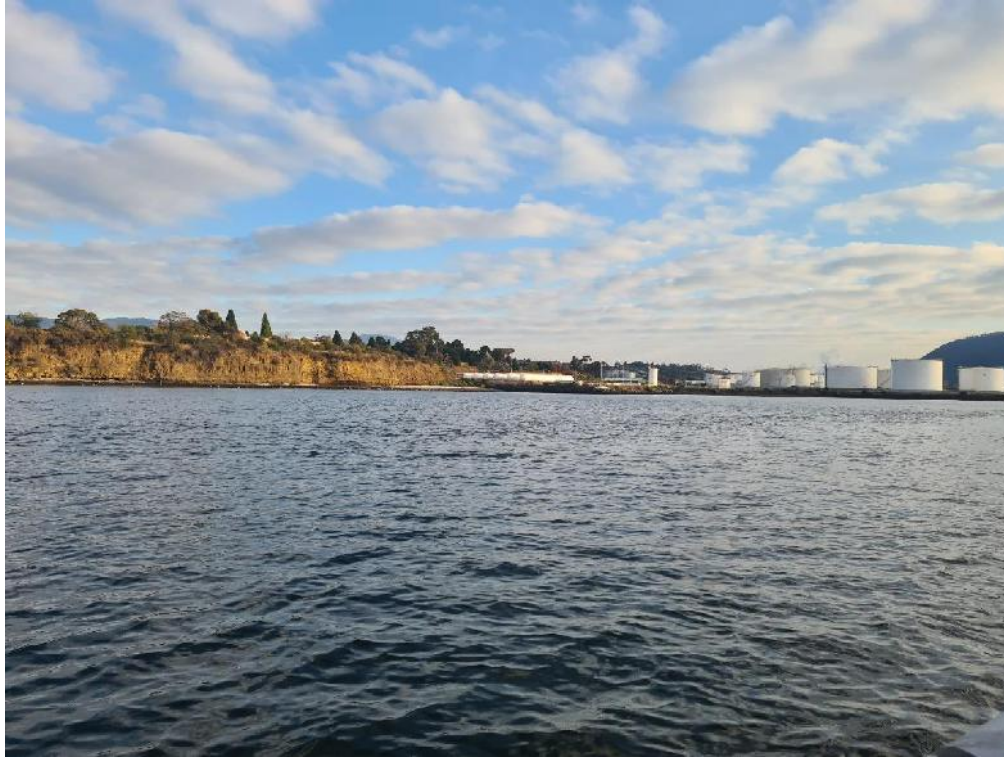
Figure 2: Existing infrastructure and shoreline near the proposed pipeline alignment.
